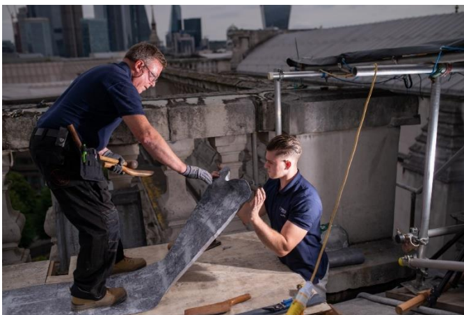
Figure: Works staff repairing the roof in early 2021.
